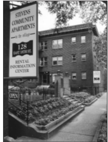
SSCO invested $500,000 of NRP funds in a $14.8 million project to renovate 618 apartments.
